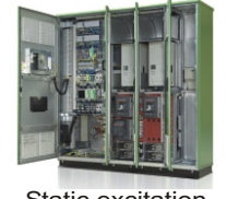
Static excitation system-UNITROL
